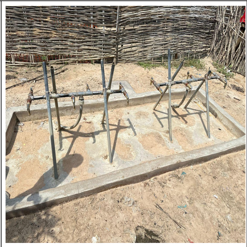
The Majook-Noon PHCC water yard at Majook-Noon Boma in Aweng showing the communal water point which currently non-functional
