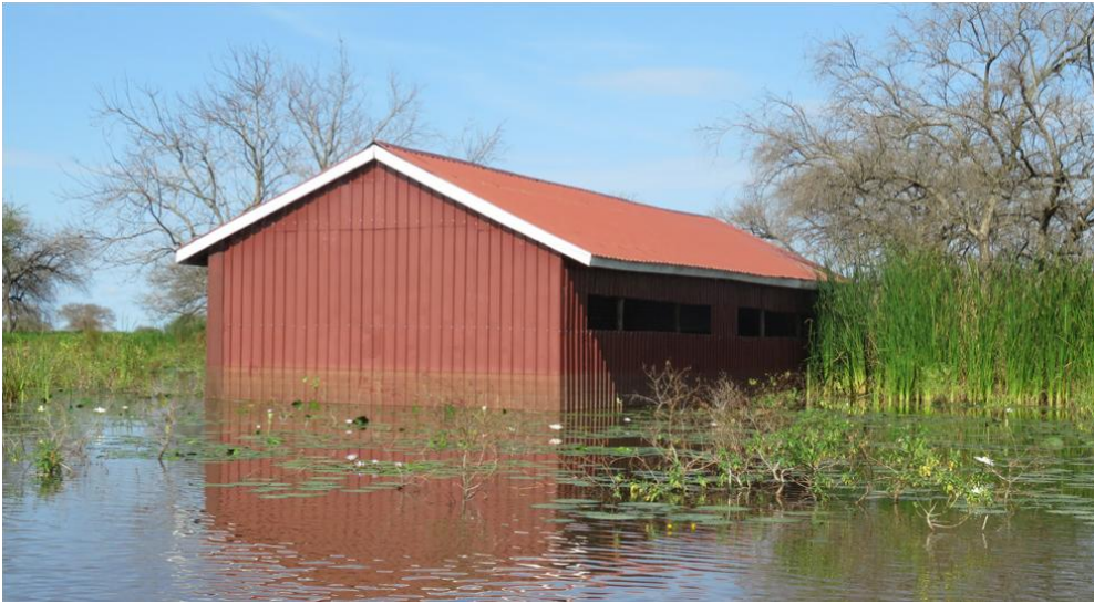
Figure 27. Flooded school in Kongor Payam © IOM 2022
