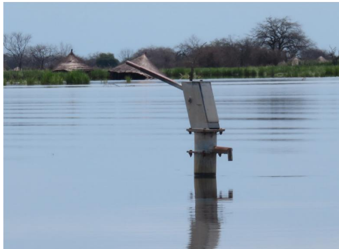
Figure 26. Flooded Borehole in Nyuak Payam
