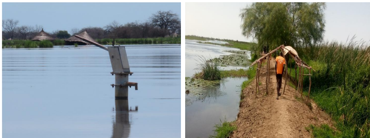
Figure 2. Photo grid showing the dike and community infrastructure that is submerged in water
