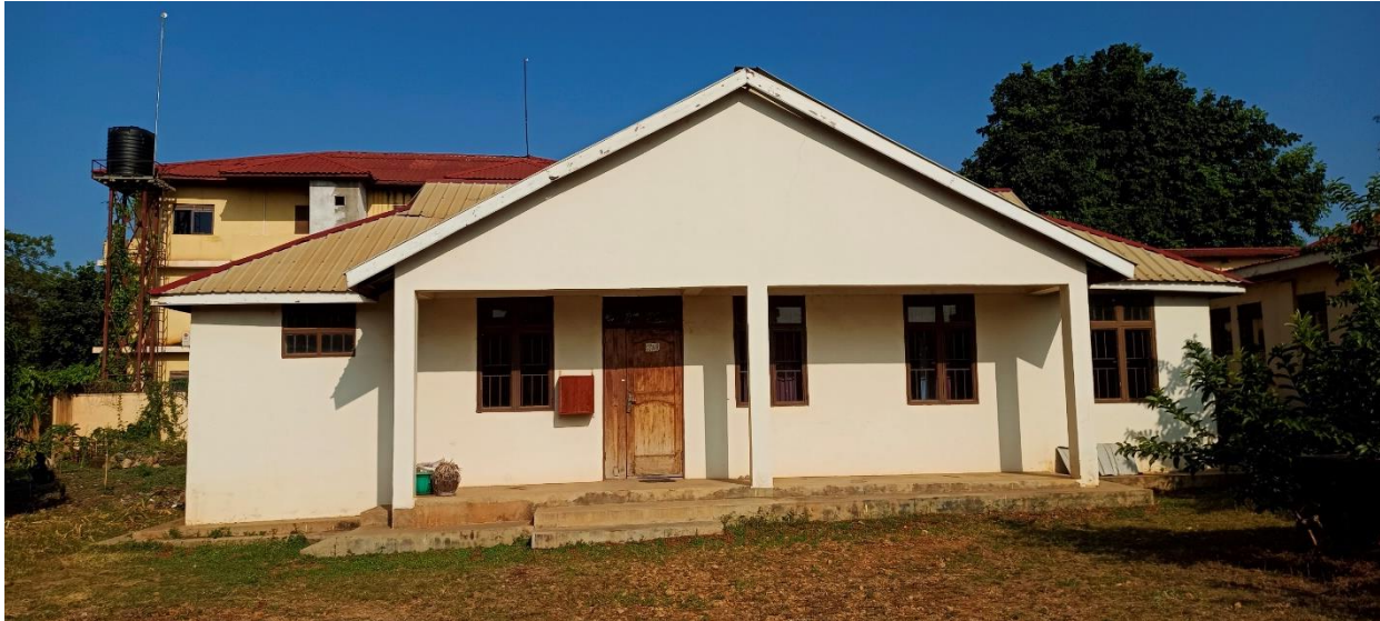
Image 1: Showing the small office block to be renovated. Image taken by Yengi Emmanuel Daro on 11-15-2022
