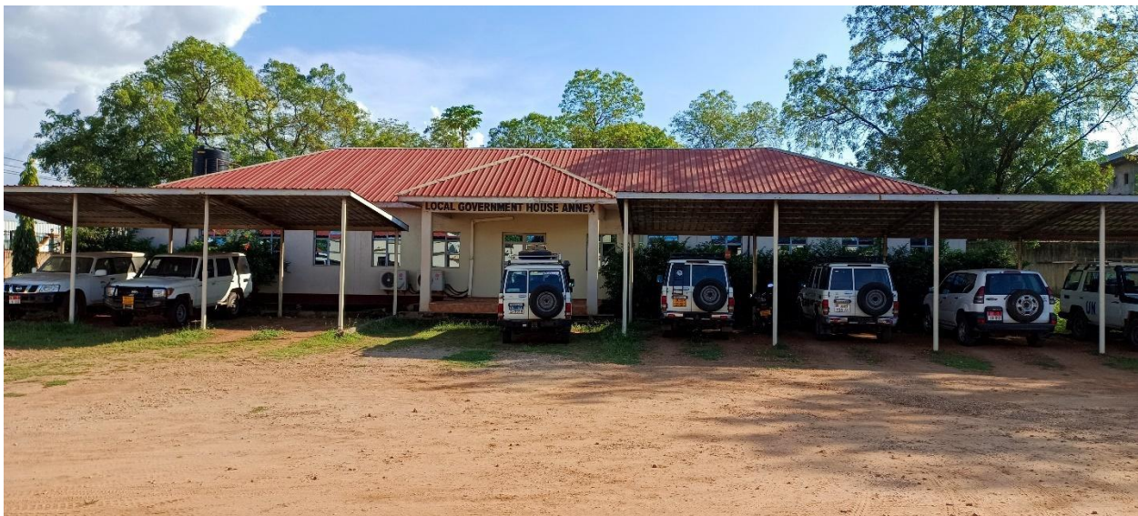
Image 3: Showing the Large office Block to be renovated. Image taken by Yengi Emmanuel Daro on 15th Nov 2022
