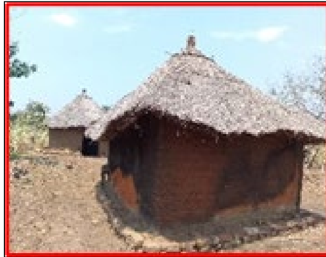
Figure 6.2-2 –Tukuls in the affected area
